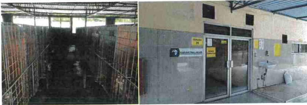
Figure 7. Final Quarantine Enclosure at Facility 1
