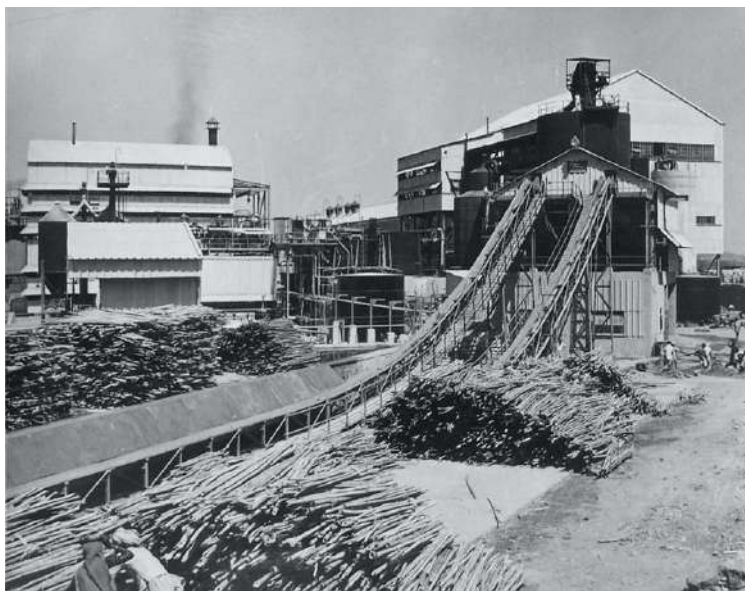
Figure 6.16. An historical photograph of the Nepa mill, showing the bamboo that supplied part of the pulp for making newspaper, with Boswellia serrata supply 60-65% of the mechanical pulp at the time (Dorset, 1970).
