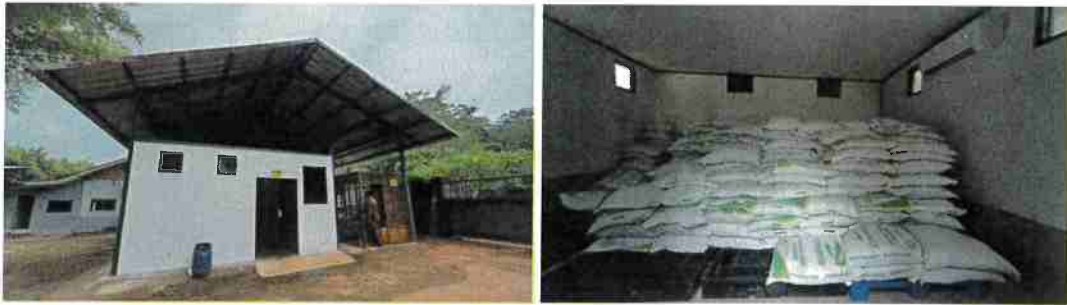
Figure 11. Feed Storage Room at Facility 1
