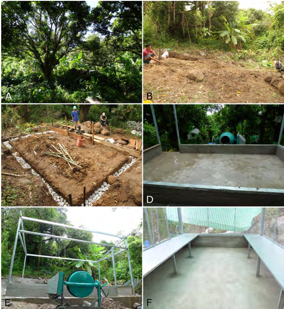
Fig. 3. Building phase 1: (A) This part of the Hon Me Station was selected for the building of the gecko house (phot. A. Rauhaus), (B) measuring and marking the cleared site, (C) starting with the fundament, (D) base plate and walls, (E) insertion of iron frames, (F) insertion of tables for the terraria. Photos: K.V. Nguyen.
