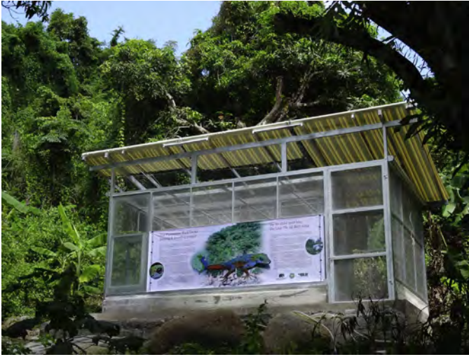
Fig. 7. The gecko house was finished in November 2014: on the top the manually adjustable rain and sun protection is visible; on the left there is the enclosure visible for visitors from outside, in the middle the weatherproof project banner, and on the right the double door system. Photo: A. Rauhaus.
