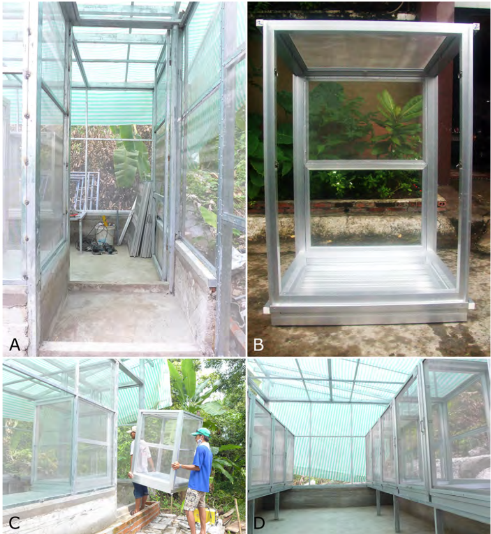
Fig. 4. Building phase 2: (A) Double door system, (B) development of the first terrarium, (C) bringing in of the terraria, (D) inside view of the gecko house with inserted terraria. Photos: K.V. Nguyen.
