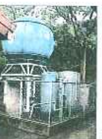
Water Filtration/ UV Light Treatment & Storage
